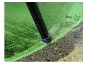
Rubber extrusion (fish bumper) after fitting
